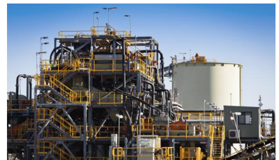
Lithium Processing Plant in Western Australia
